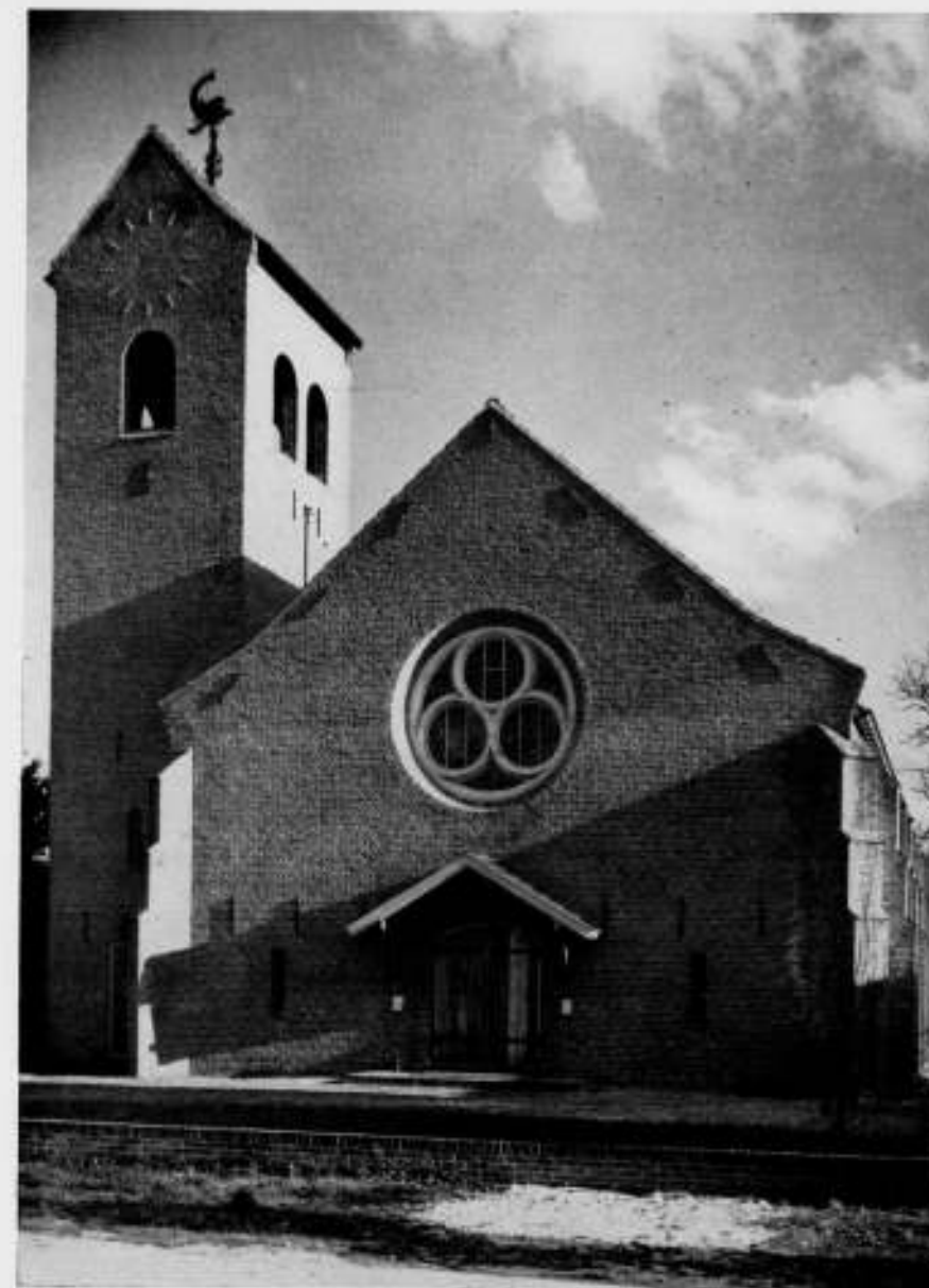
NED. HERV. KERK TE COLMSCHATE. ARCHITECT W. VERSCHOOR.
