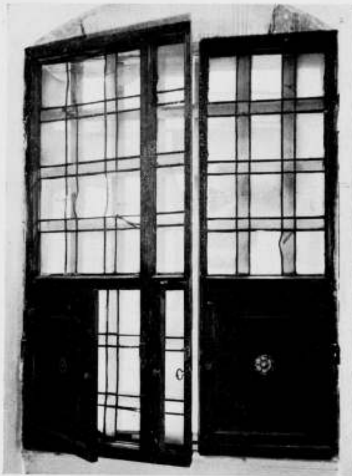
FIG. 8. ORIGINEEL VENSTER IN DEN SOKKEL.
